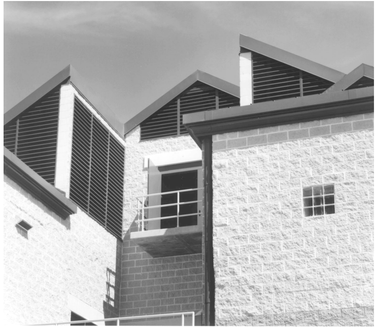
Custom Louver Installation
